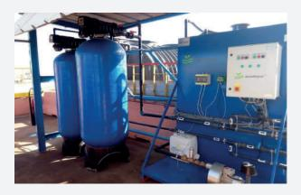
The treatment and reuse of Wash Water involves a series of in line treatment procedures in order to achieve the required quality for washing operations.
